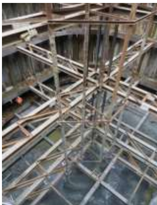
Figure 2. Picture of the trial pit in Antwerp (Belgium).
