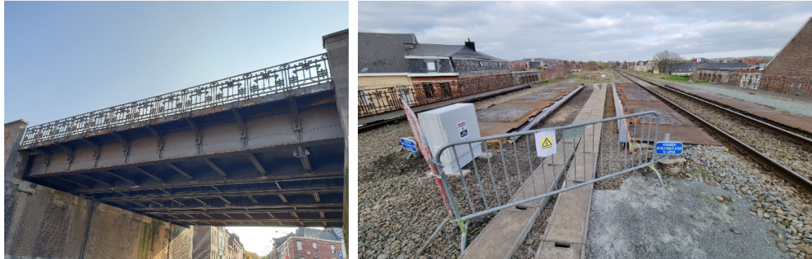
Figure 101. The Nieuwebrugstraat bridge, as seen underneath (left) and from the top (right).
