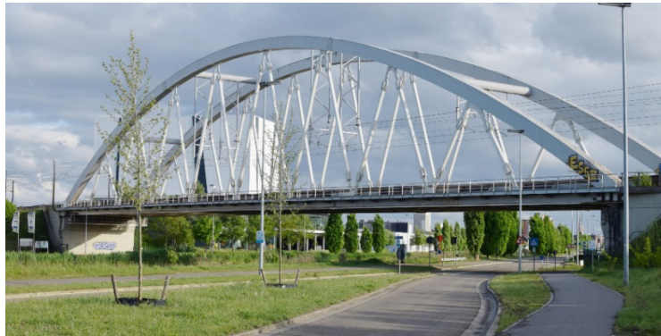
Figure 98. The KW51 bridge, as seen from its north side. Photo reproduced with permission from [25].
