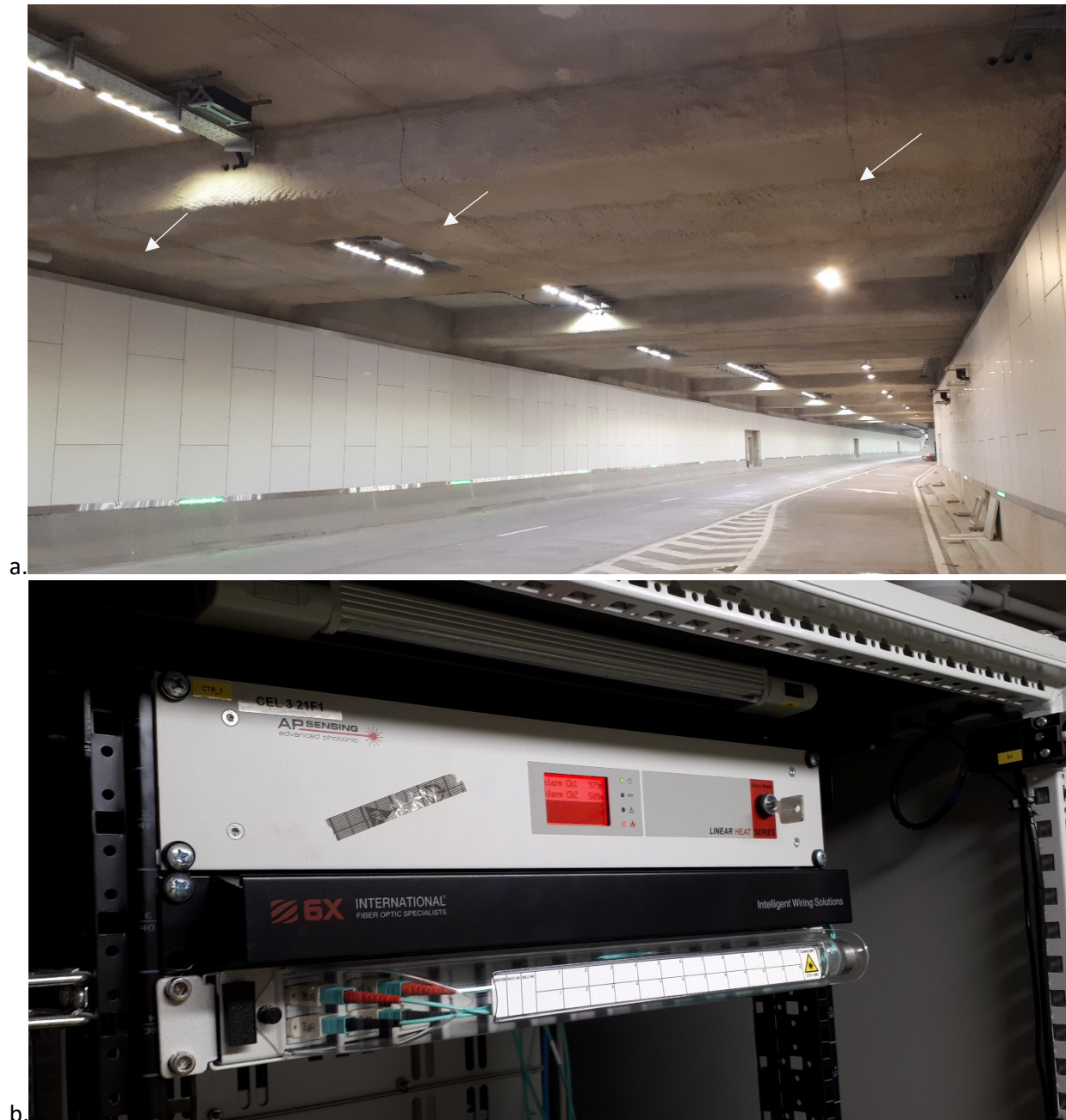
Figure 121. (a) Above each lane, a temperature sensing cable is mounted on the tunnel ceiling. (b) One of the two installed DTS units, installed in a network cabinet.
