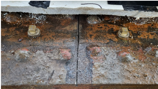
Figure 103. Chainsaw cut at the middle of the monitored span of the Nieuwebrugstraat bridge. The optical fiber that monitors this part of the bridge can be seen, attached to two clamping blocks. An FBG sensor exists in between the two clamping blocks.
