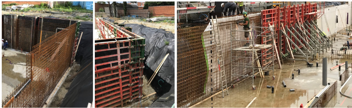
Figure 79. Two of the monitored basements walls. (left) Basement with a double formwork with pins to connect the two sides. (right) Basement cast in front of a Berliner wall with a traditional formwork closing off the other side.
