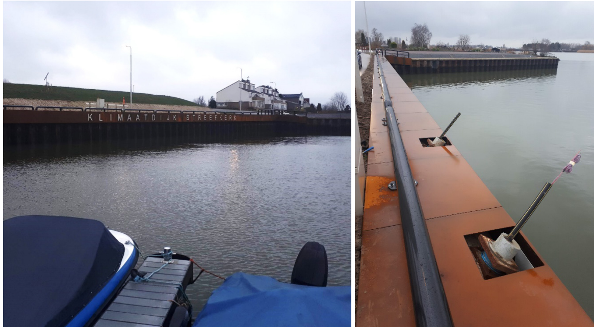
Figure 113. View of the project location after finishing the dike reinforcement and the new quay wall. The black tubes extending from the anchor heads were used for water pressure measurements, which were converted into a vertical displacement profile.
