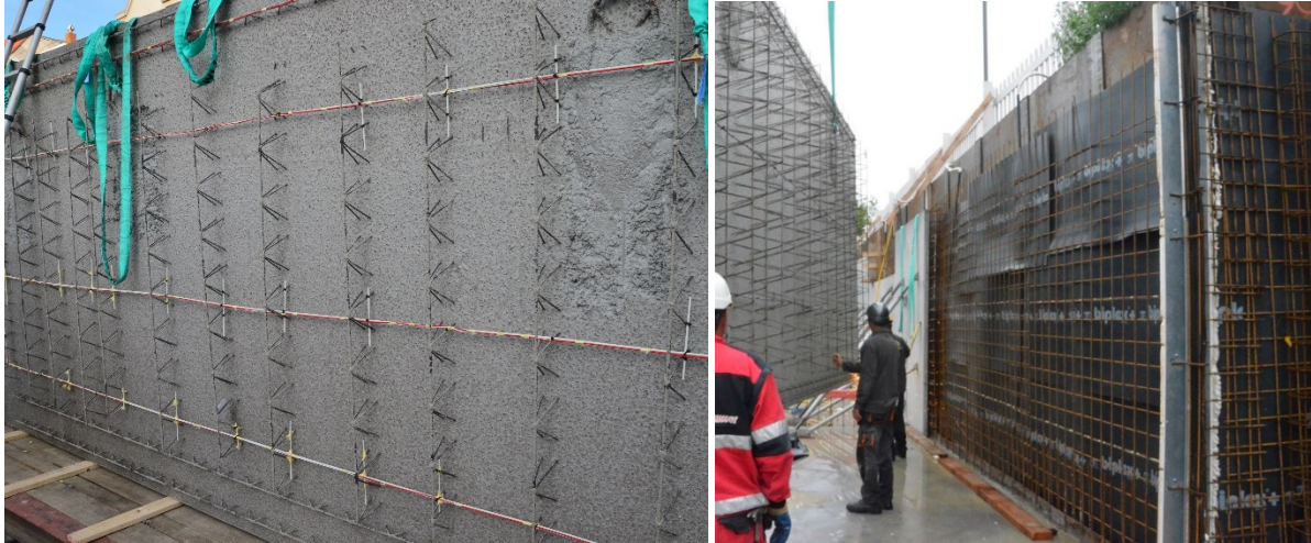
Figure 87. (left) First layer of optical fiber sensing cables attached with support rods to the precast concrete shell. (right) View of the optical fibers installed on the reinforcement mesh at the rear of the concrete core, before closing the wall with the precast concrete shell.
