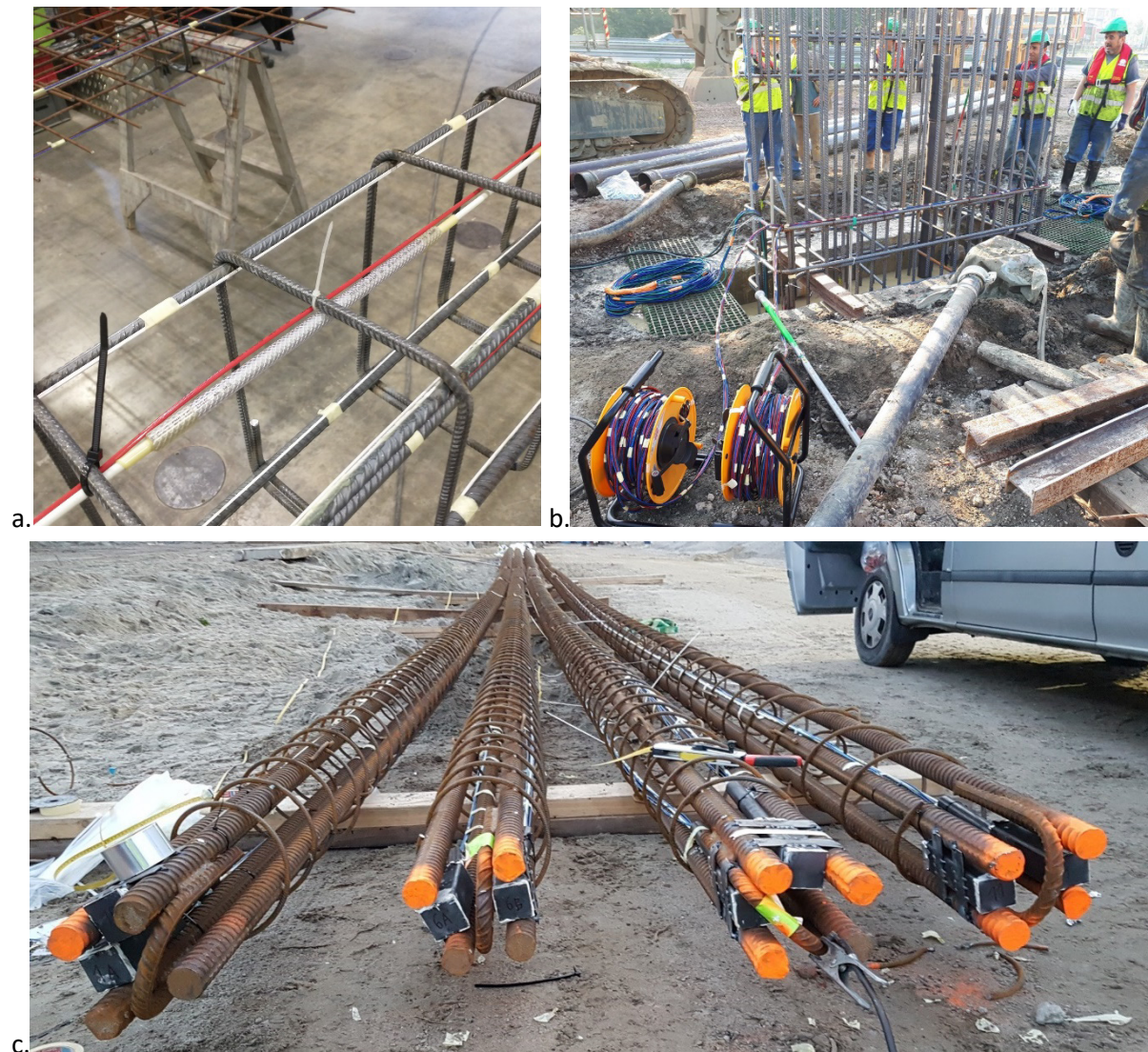
Figure 51. Examples of integration of the fiber optic cables directly in the structure. In all these cases, the fibers are attached to the reinforcement cage of the concrete beam (a), of the diaphragm wall (b) and of the foundation pile (c).
