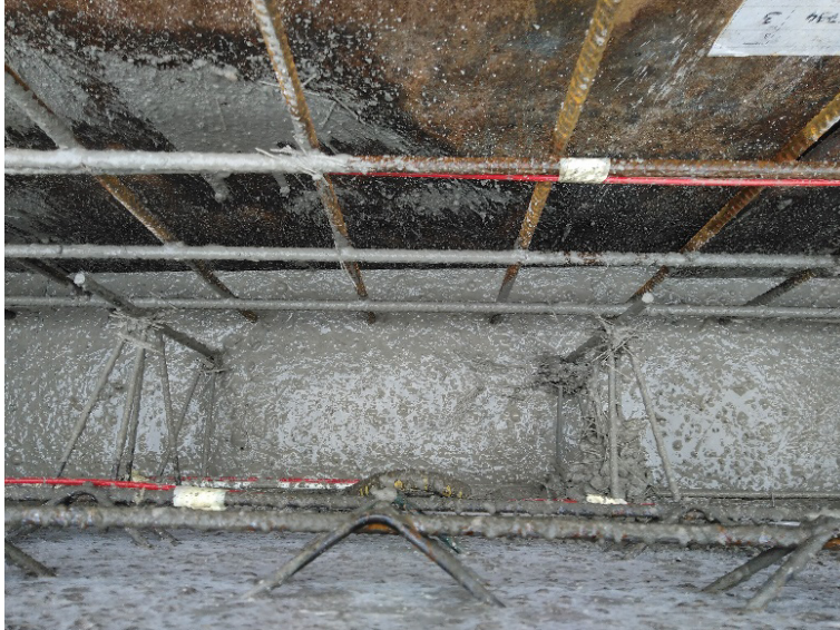
Figure 86. Cast-in-place concrete core poured on site between the precast panel and in this case a Berliner wall.
