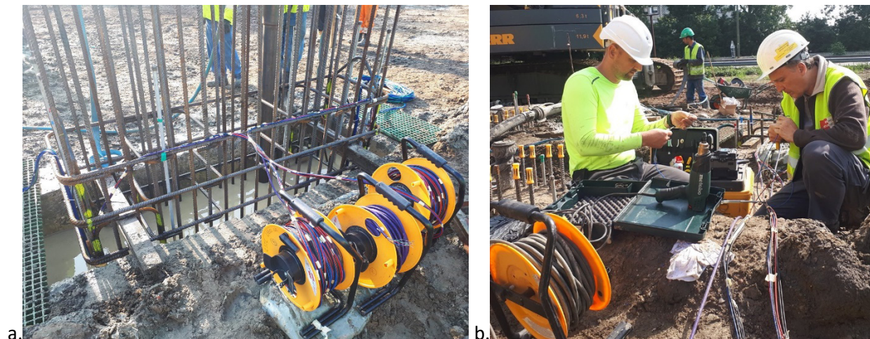
Figure 124. (a) Sensor cables during the lowering of the reinforcement cage in the excavated panel. (b) Splicing of the sensor cables prior to concreting the diaphragm wall panel.
