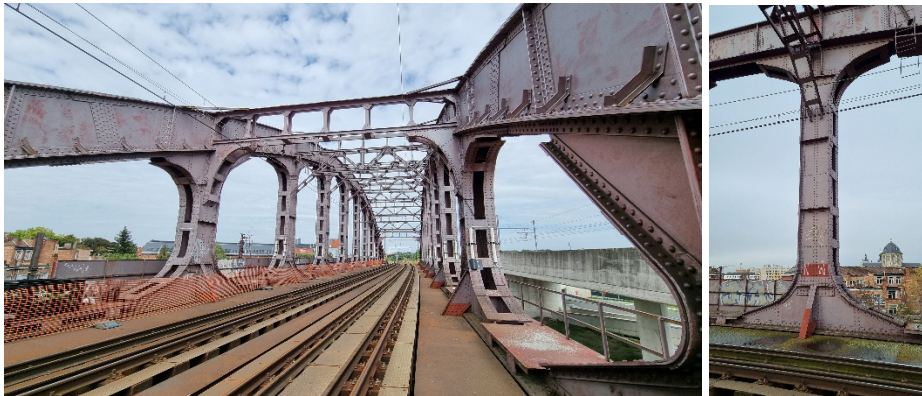
Figure 105. The Vierendeel bridge over the Leuvensesteenweg, as seen from its west side (left) and one of the north columns (right).
