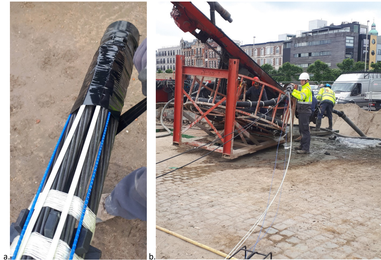
Figure 123. (a) Attaching the distributed strain sensing cables to the bottom of the steel tendons of a ground anchor. (b) During installation of the ground anchor in the borehole. Simultaneously, the fiber optic cables are integrated.
