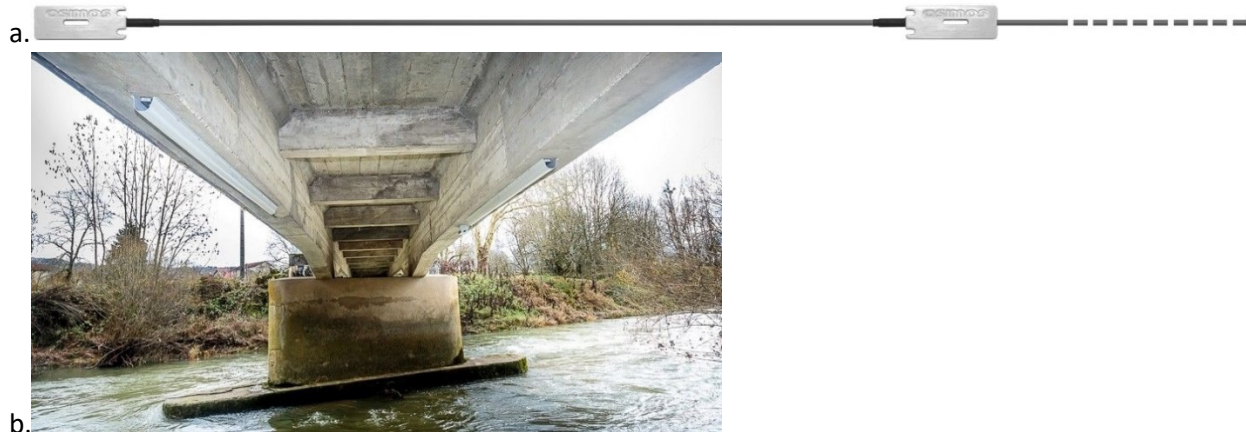
Figure 36. (a) Illustration of the OSMOS optical strand to measure elongation. Standard measurement base of 1 and 2 m. (b) The strand attached to the bottom of reinforced concrete bridge. Source: www.osmos-group.com .
