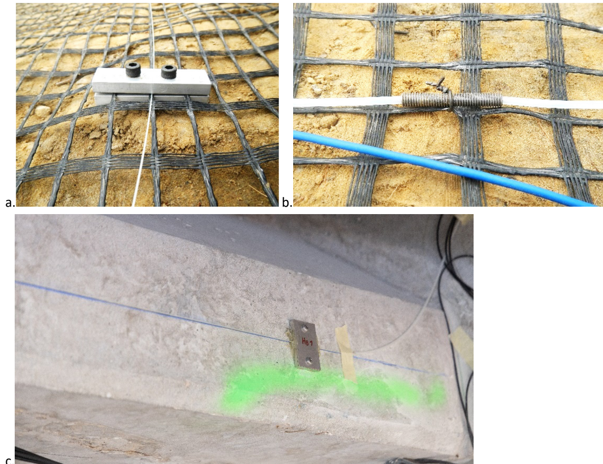
Figure 49. Examples of mechanical fixation of sensing fibers.
