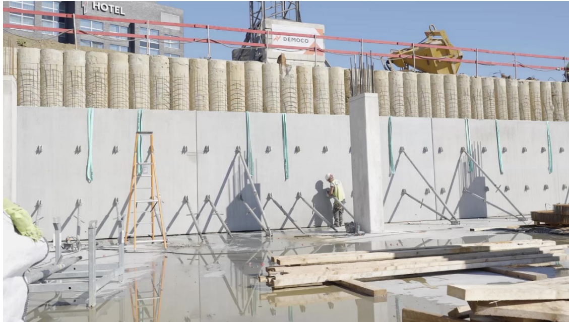
Figure 85. Single-sided precast concrete twin wall system developed by Prefaxis, for realising basement walls against an earth retaining structure.
