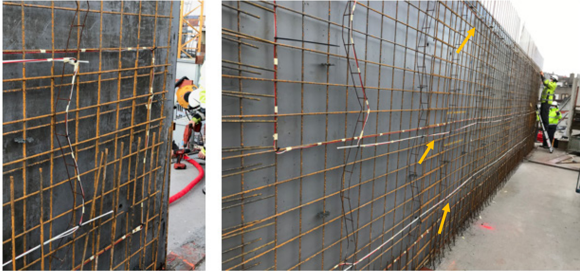
Figure 80. Illustration of the typical monitoring setup used in the REINFORCE project. With optical fiber sensing cables at 3 levels and 2 depths in the wall (indicated with the yellow arrows).
