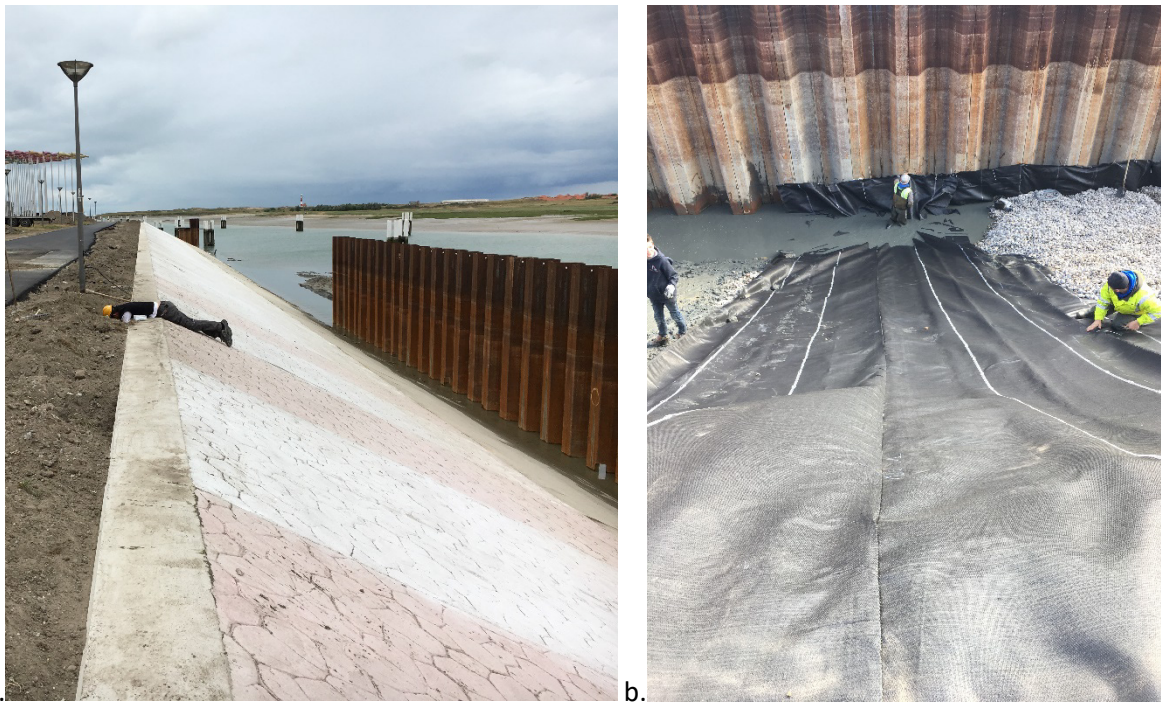
Figure 96. (a) The finished dike slope in the harbour channel of Nieuwpoort, Belgium. (b) The geotextile during instrumentation with fiber optic FBG sensors.
