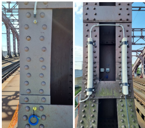
Figure 107. Installation of the optic fibers: (left) clamping blocks for connecting a glass fiber to a column of the bridge; (right) thermal insulation covering fiber and clamping blocks.
