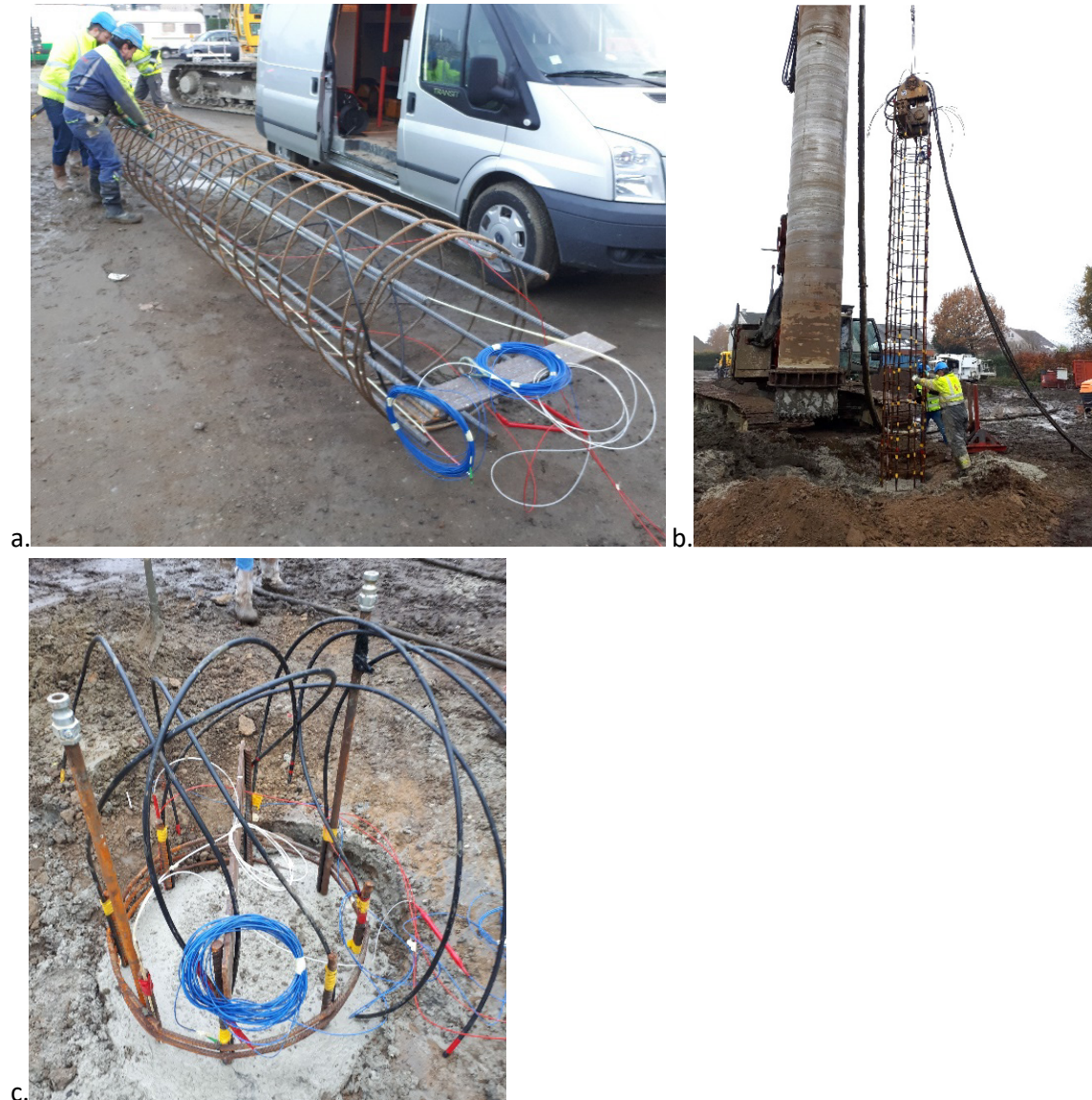
Figure 122. (a-c) Instrumentation of the reinforcement cage of a CFA foundation pile, before, during and after execution.
